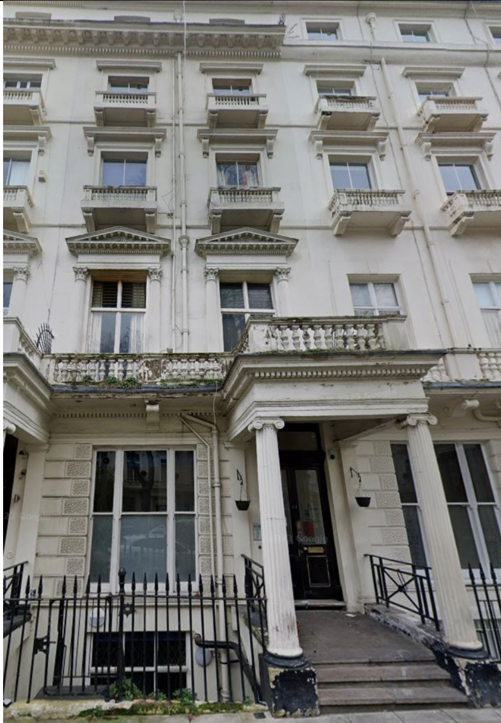
Photograph of front of the building
