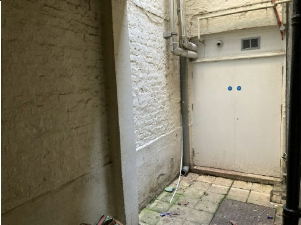
View within courtyard where the 5 air source heat pumps will be located
